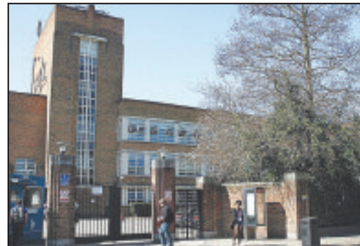
Scheme: Plans for a new educational centre have been agreed for the Richmond College site in Egerton Road
